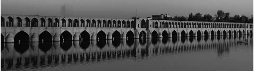
Si-o-se Pol Bridge, Isfahan, Iran
